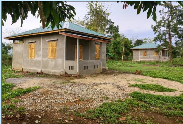
Construction of 19 low-cost houses in Da Lau Gyi, Myitkyina Township
