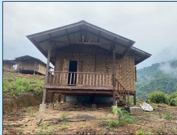
Construction of houses in Yit Kyaw village, Chi Phwe Township
