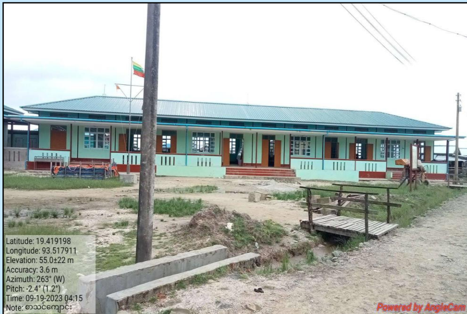
School Building No. 1
