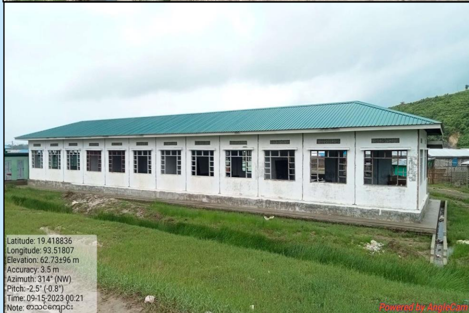
School Building No. 2
