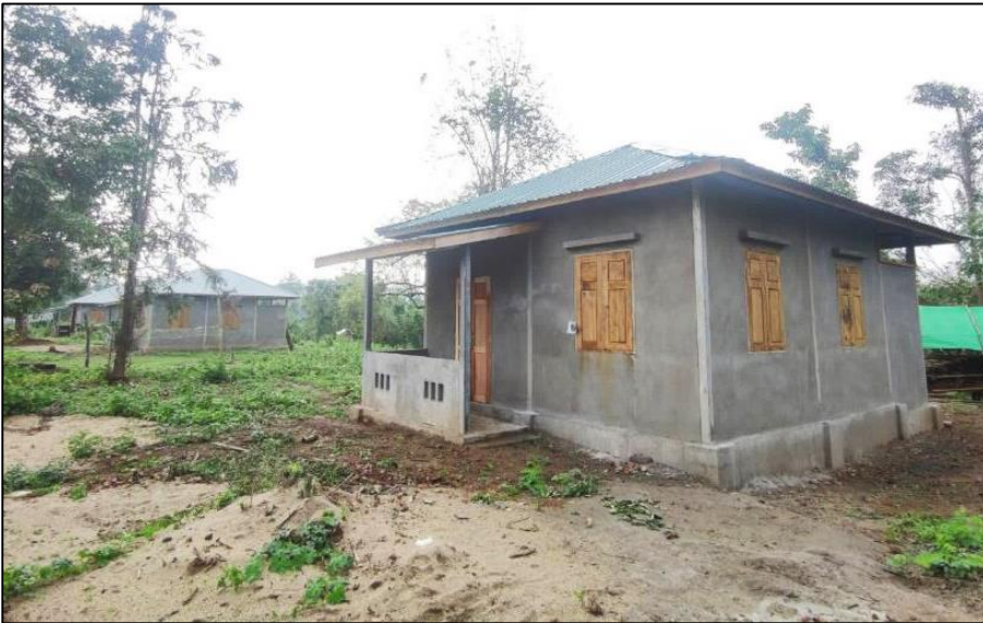
Construction of low-cost houses in Dabang Yang, Waingmaw Township
