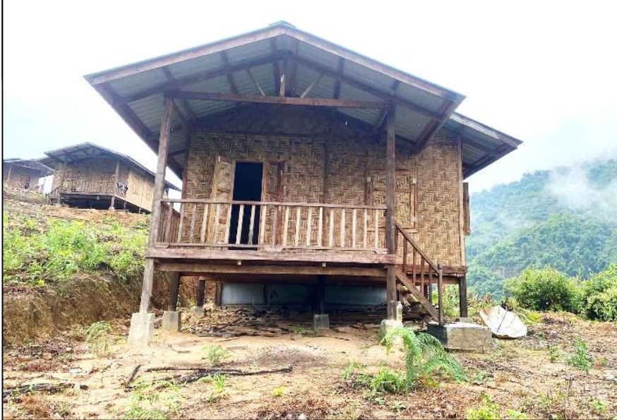
Construction of houses in Yit Kyaw village, Chi Phwe Township
