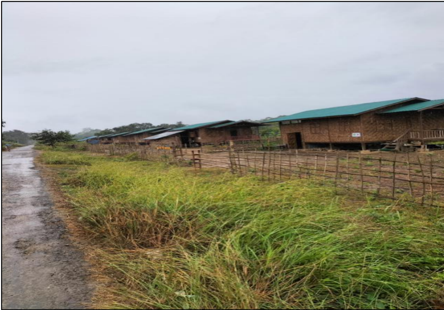
Construction of houses in Ye Kyi village, Myitkyina Township
