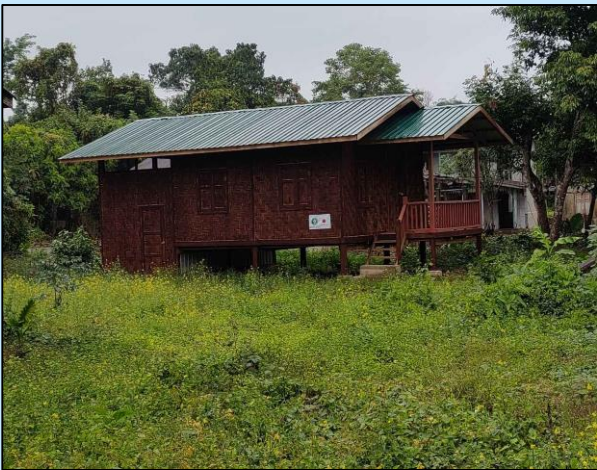
Construction of houses in Gara Yang village, Waingmaw Township
