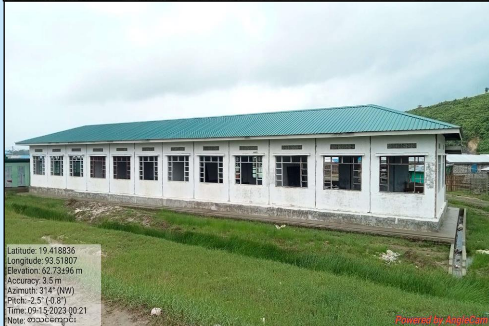
School Building No. 2
