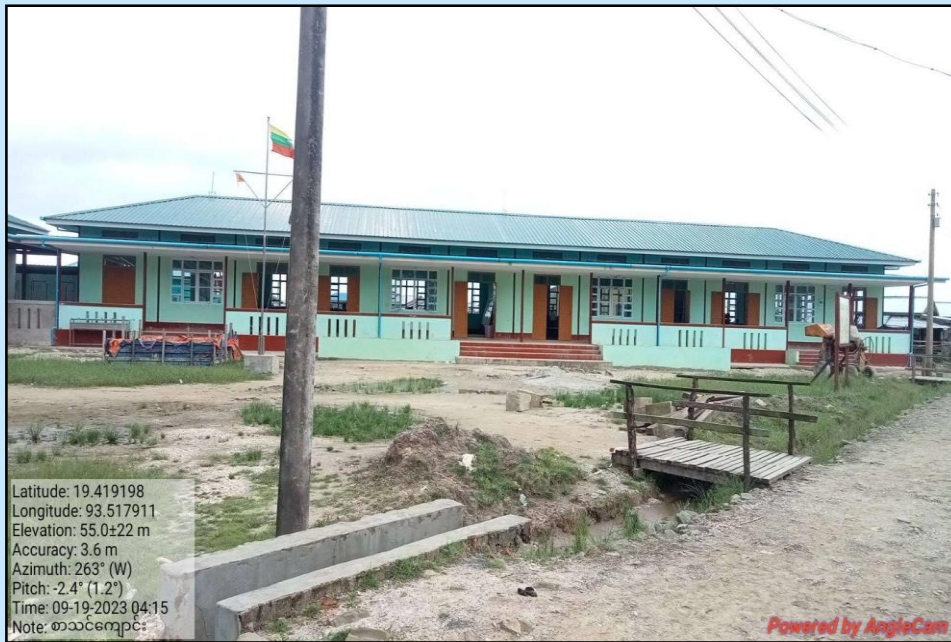
School Building No. 1
