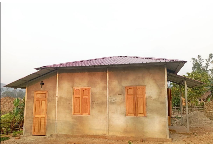
Construction of low-cost houses in Nansanyan, Waingmaw Township
