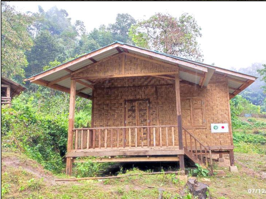
Construction of houses in Jingloi village, Chipwe Township
