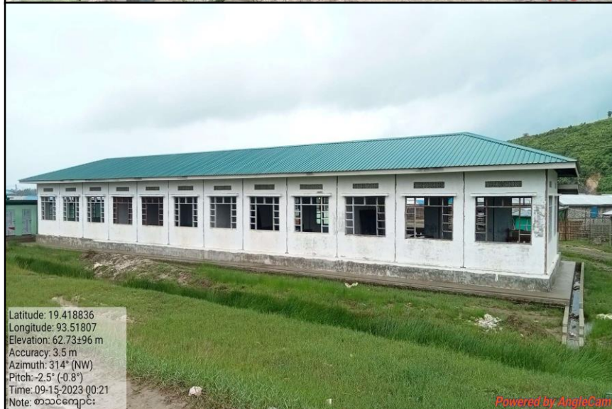
School Building No. 2
