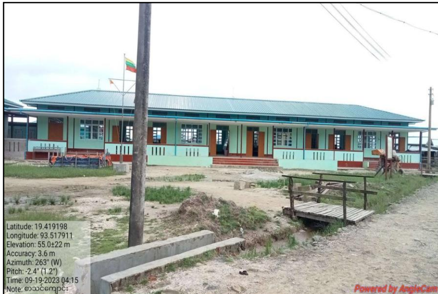
School Building No. 1
