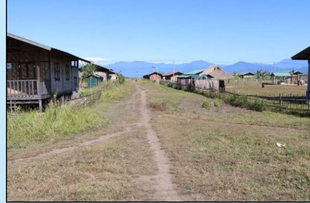
Construction of houses in Zeedan (2) village, Putao Township
