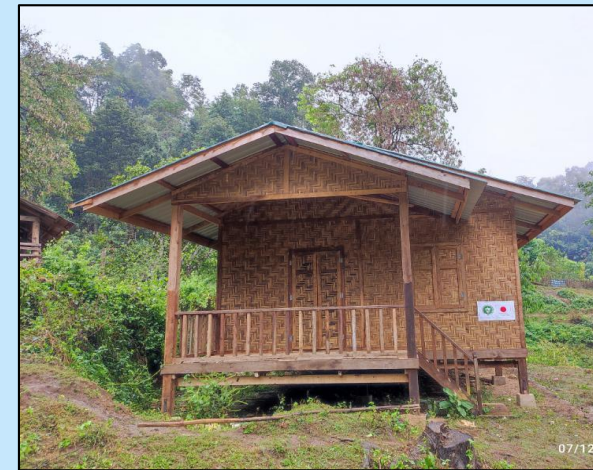
Construction of houses in Jingloi village, Chipwe Township
