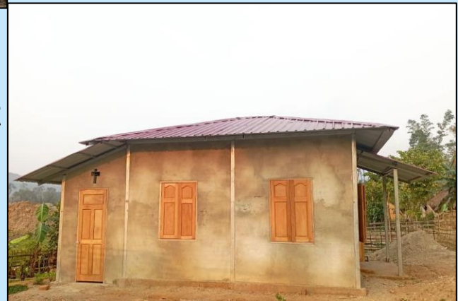
Construction of 39 low-cost houses in Nansanyan, Waingmaw Township
