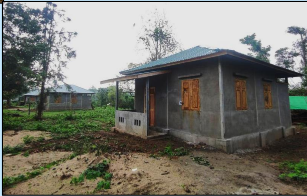
Construction of 30 low-cost houses in Dabang Yang, Waingmaw Township
