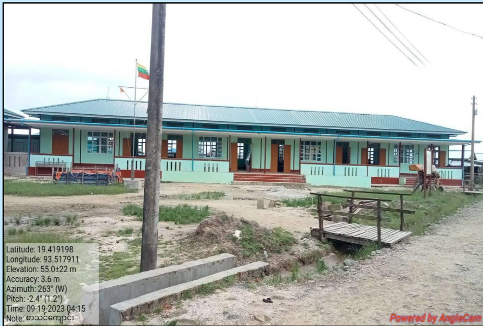
School Building No. 1
