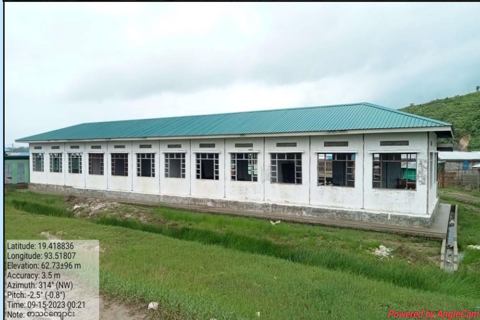
School Building No. 2
