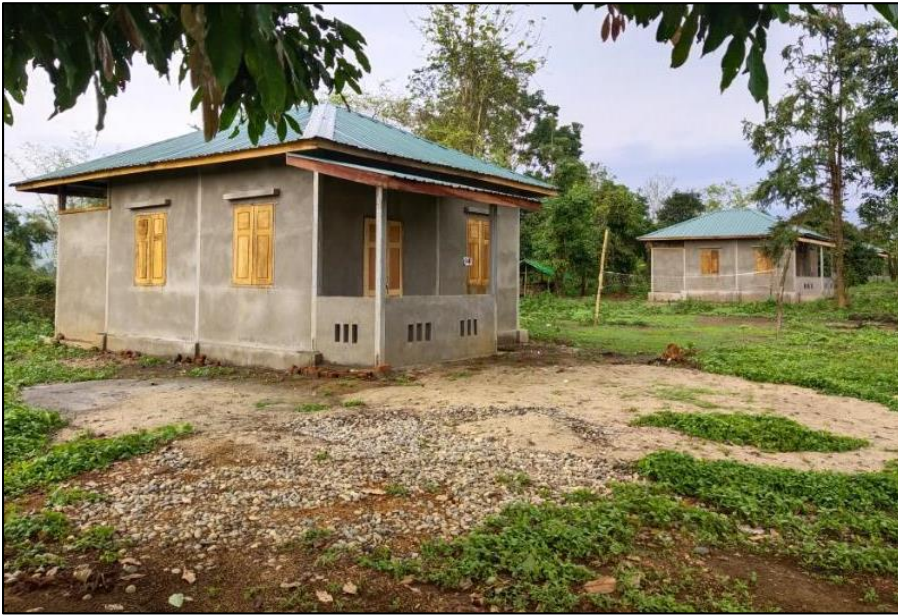
Construction of low-cost houses in Da Lau Gyi, Myitkyina Township
