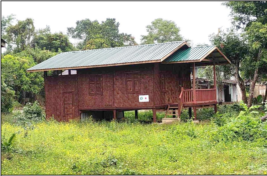
Construction of houses in Gara Yang village, Waingmaw Township
