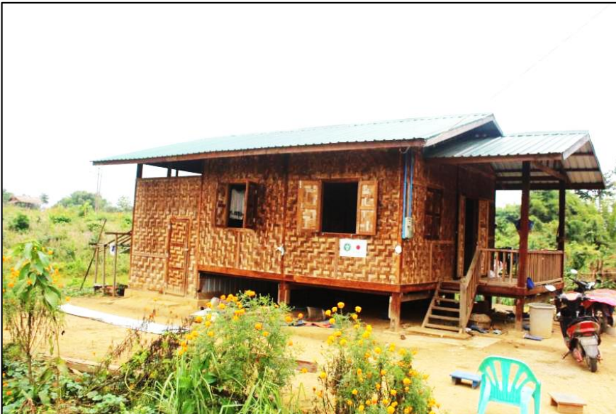
Construction of houses in Garayang village, Mansi Township
